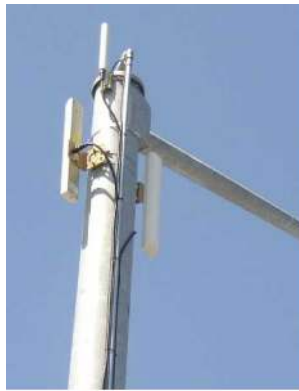
Figure 3. Example of Antenna Installation on Light Pole
