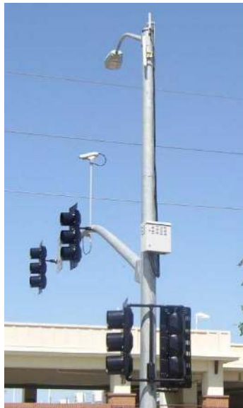
Figure 3. Example of Antenna Installation on Light Pole
