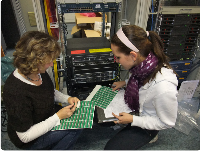
Highway Authority employees benefit from greatly simplified maintenance and improved control options.
