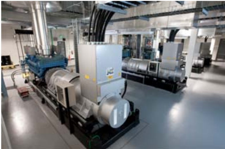
Figure 6. Rotary Uninterrupted Power Supply (UPS) systems in Allen, Texas Data Center
