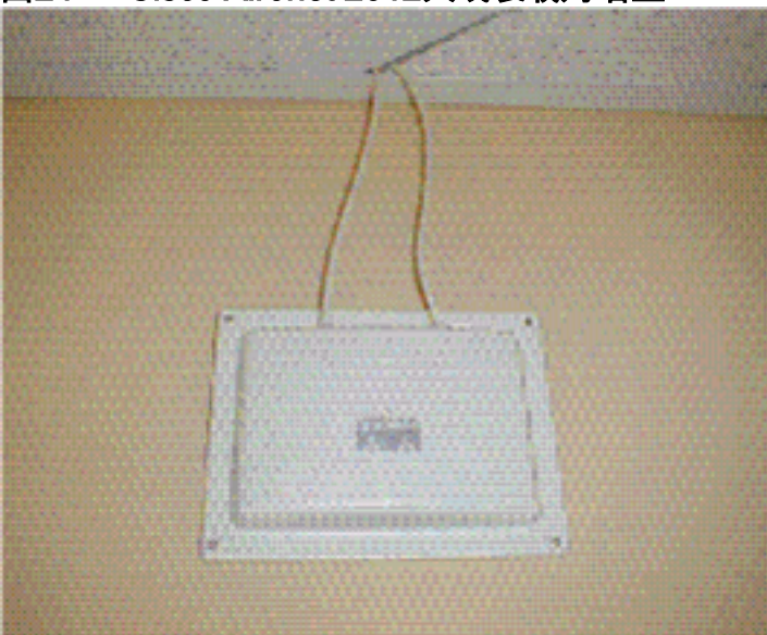
图24 — Cisco Aironet 2012天线装载对墙壁
