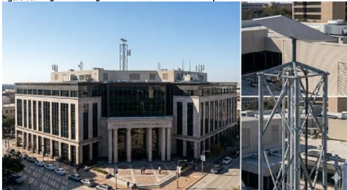
Figure 16. Regional banking hub with mast mounted Starlink performance terminals
