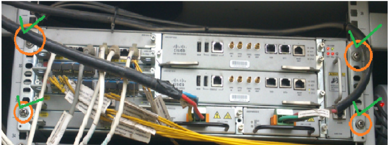
Figure 6: Securing the Router with Screws
