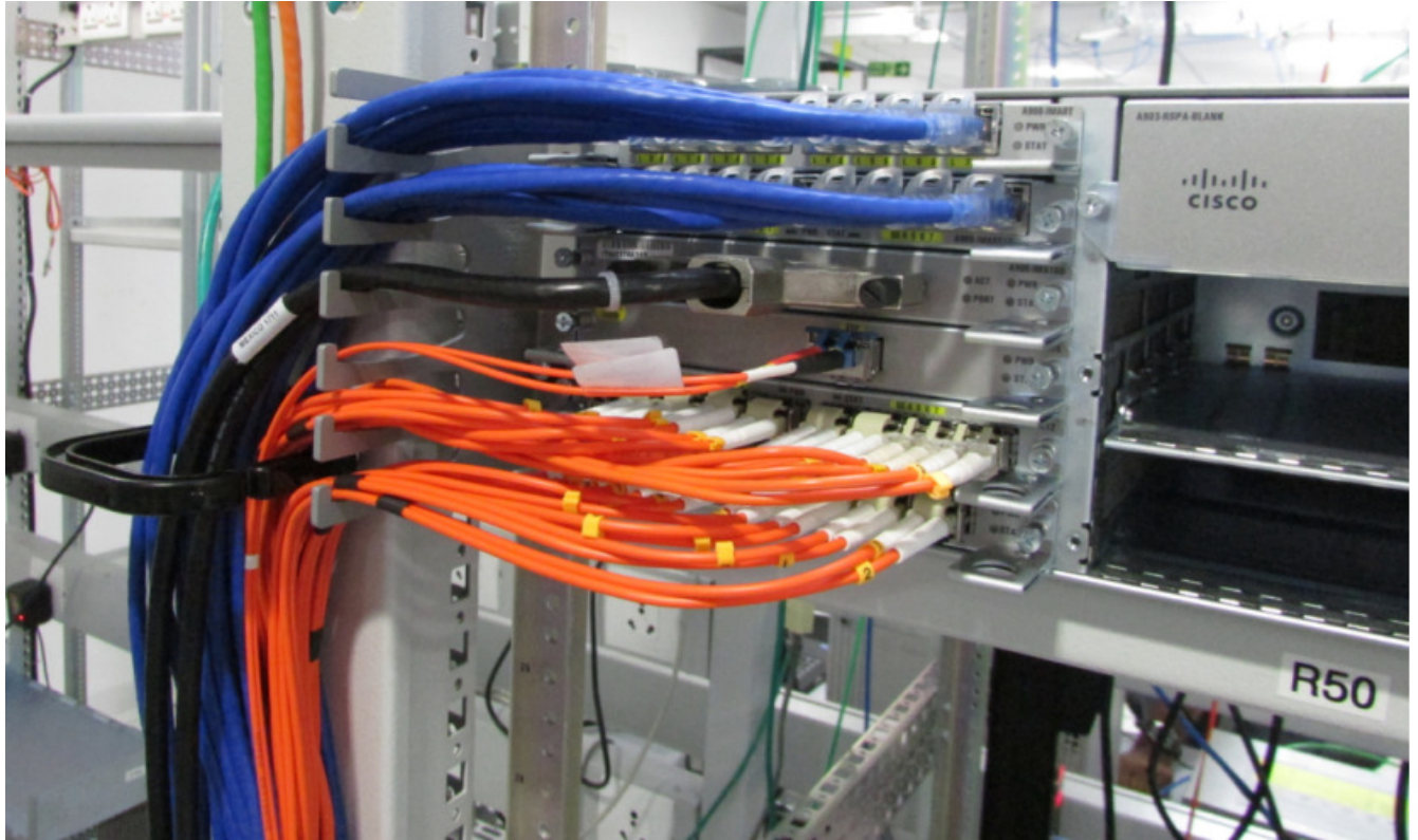
Figure 2: Using Cable Management Brackets
