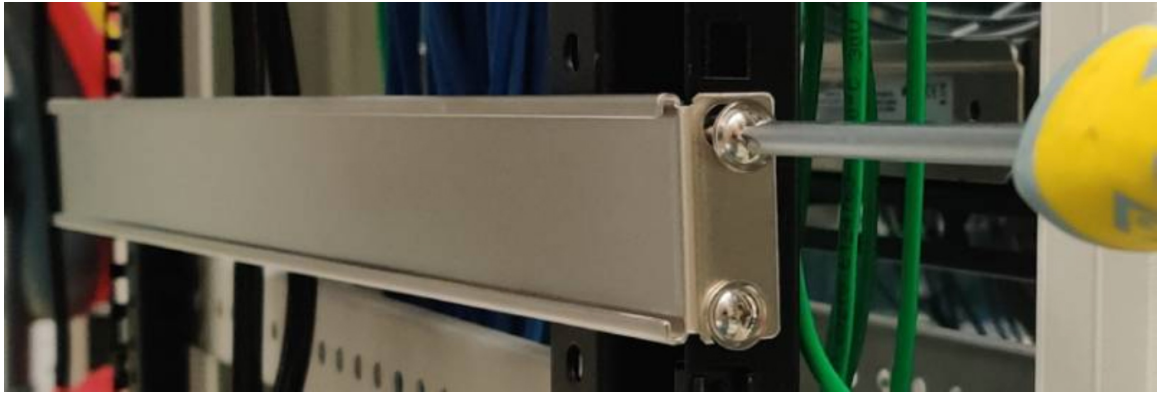
Figure 2: Attaching the left hand side rail.
