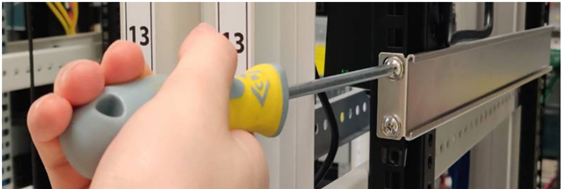
Figure 2: Attaching the left hand side rail.
