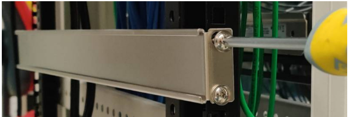
Figure 7: Attaching the right hand side rail.
