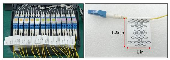
For labelling of front cables patched to the cassette, a flag label can be used. This label should be attached at the end of the boot. Kindly refer to the following suggestions for labelling sizes:
