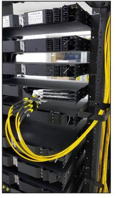
**4.3.1.3.** Route and connect the MPO cable to its terminating end.
