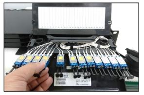
**5.1.7.** Remove the dust caps to insert the connectors to the LC/UPC simplex adapters. Carefully hold the cassette adapter holder then simply pull out the dust cap.
