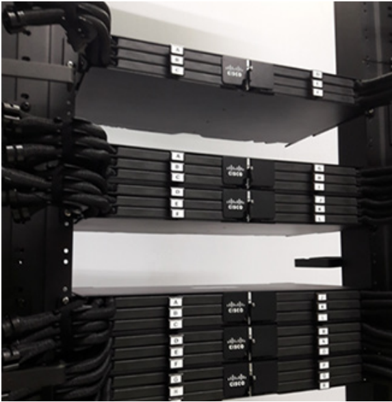
Figure 1. Cisco's 1RU, 2RU, and 3RU SMF and MMF panels
