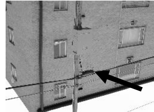
Standby (battery backup) line power supply
