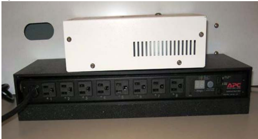
Figure 1-6 Place Isolation Transformer on the Rack
