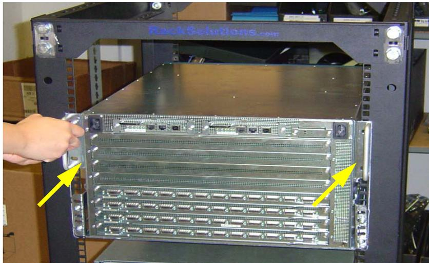
**Figure 2-12:** Screw Handles to the Rack Posts
