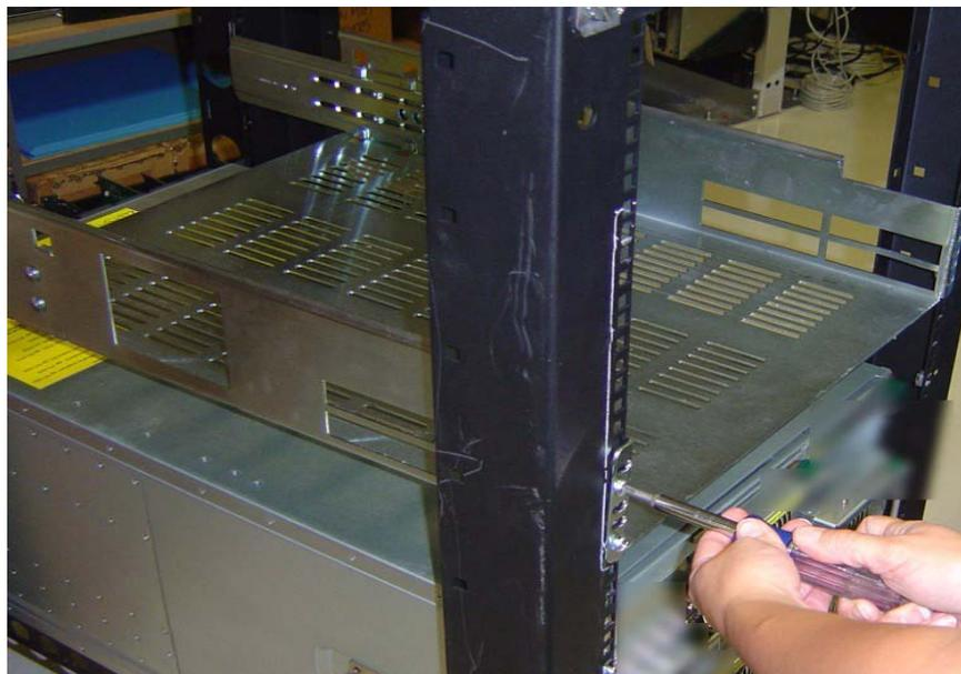
**Figure 2-9:** Screw the Shelf Ears to the Rack Posts
