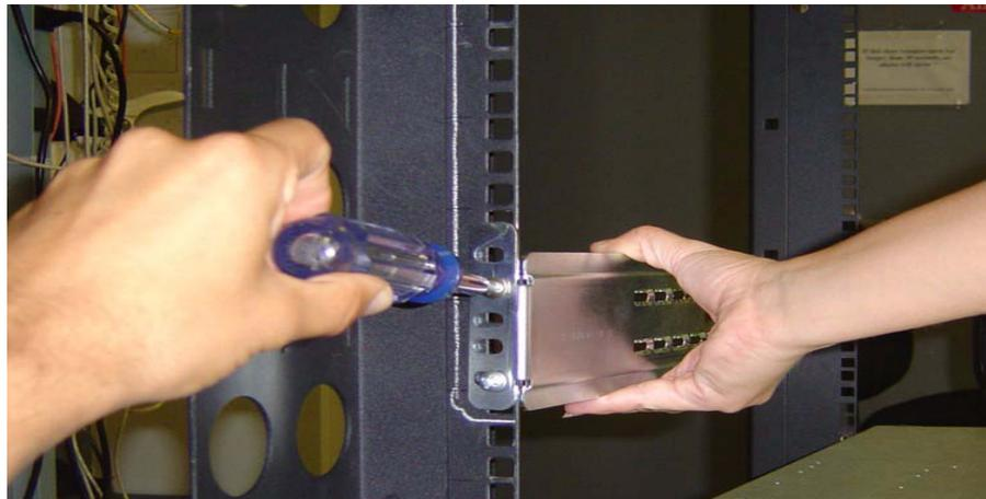
**Figure 2-5:** Attach Brackets to Post Separate from Shelf Unit
