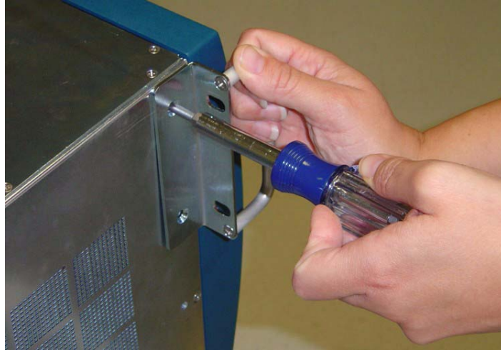
Figure 2-1: Install the Rack Ears on the Chassis
