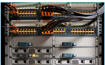
Lowers costs with 239 virtual servers operating on just 5 server blades
