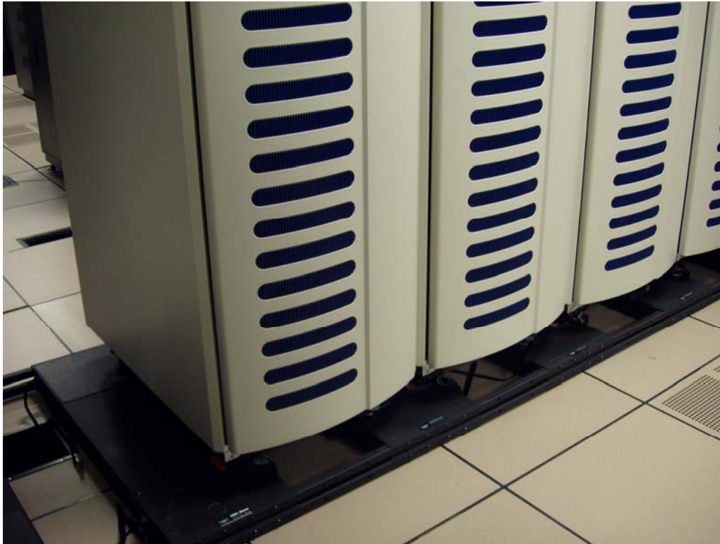
Figure 6. Servers on Seismic Isolation Platforms
