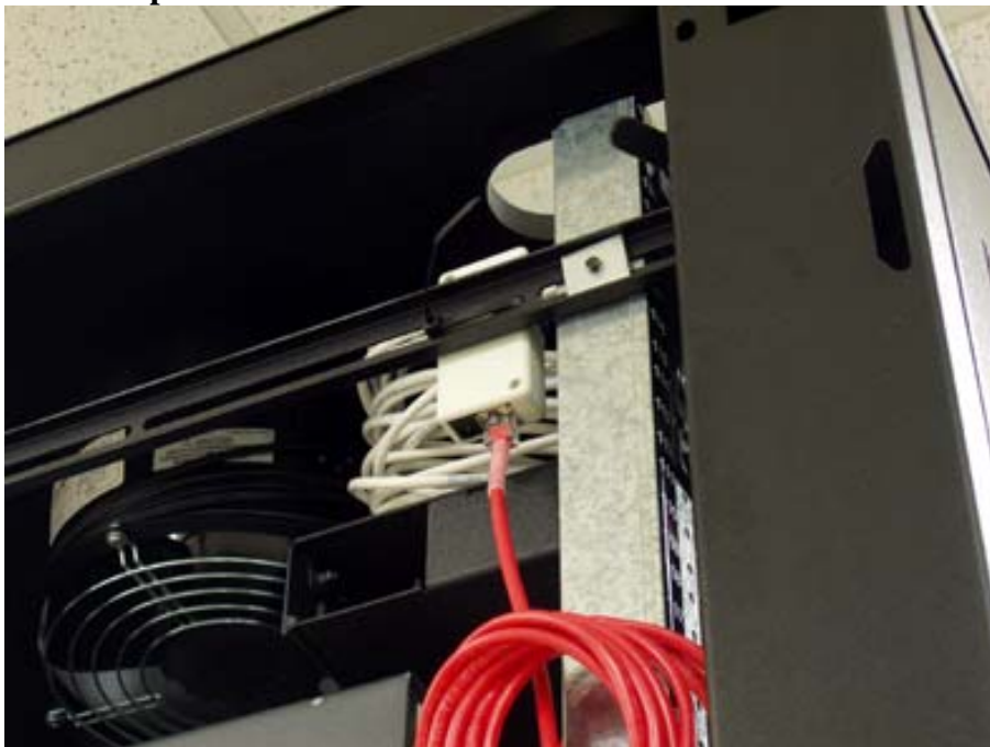
Figure 1. Temperature Sensors in a Rack
