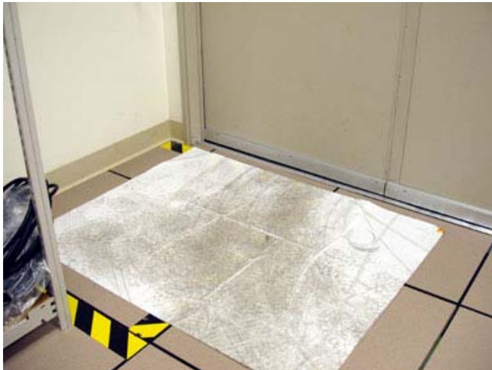
Figure 5. Sticky Dust-Trapping Mats in the Doorway
