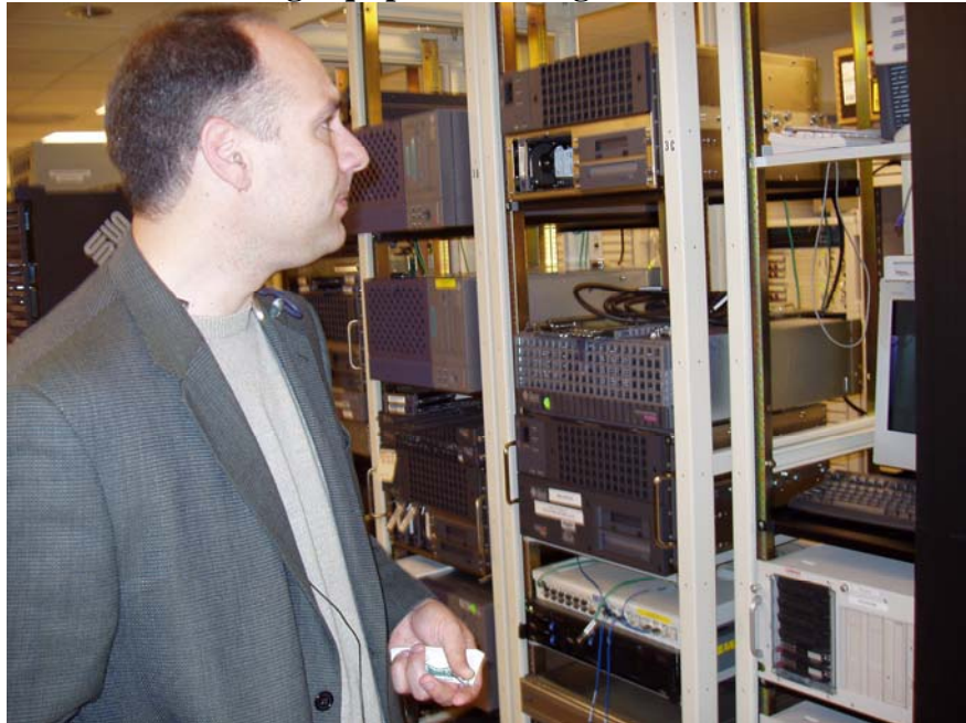
Figure 20. Dick Reviewing Equipment Changes in the Build Room
