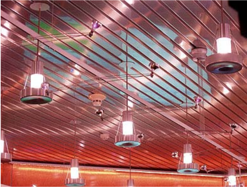
Figure 6. Ceiling Lighting in the OCC
