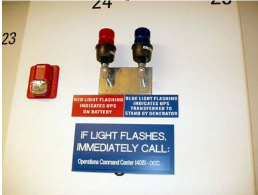
Figure 34. Red and Blue Generator lights
