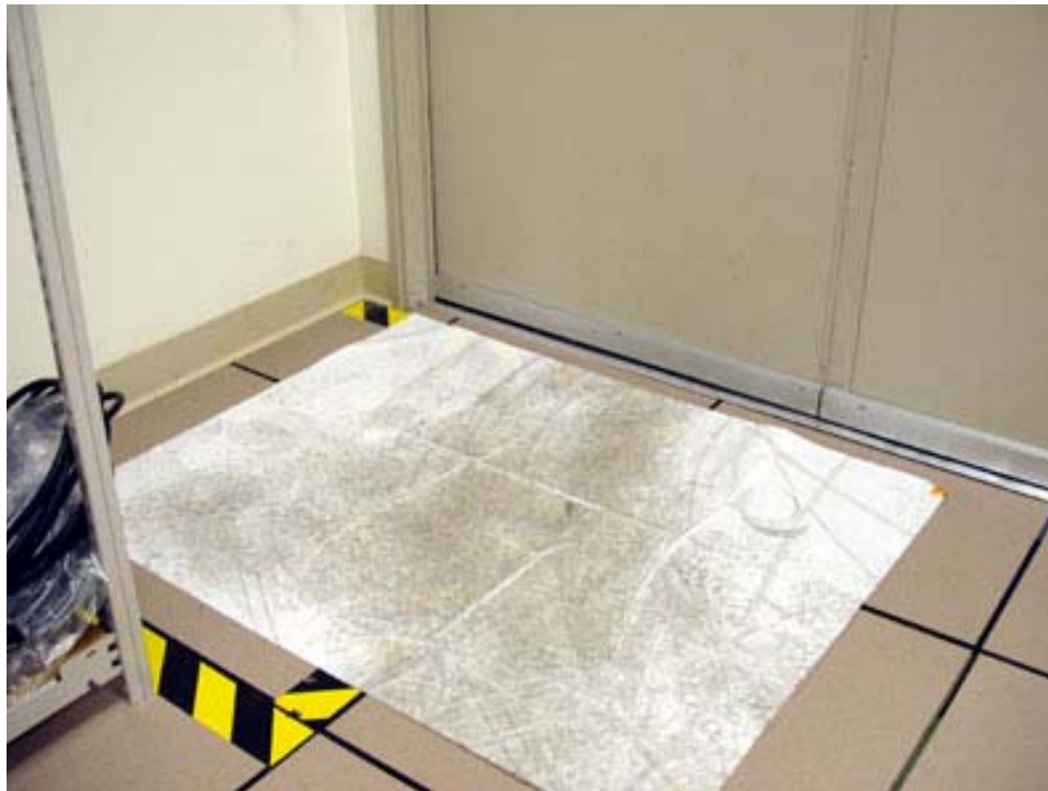
Figure 42. Sticky Dust-Trapping Mats in the Doorway
