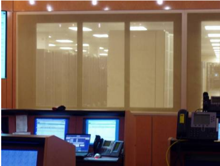
Figure 21. View of the Data Center from the OCC Window
