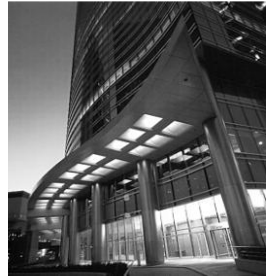
Fujitsu Headquarters Tokyo, Japan
