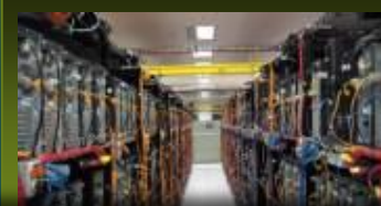
Complex Provisioning, Silos
