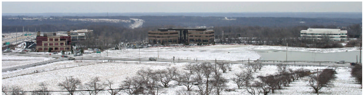
Figure 18. It is easy to link any or all of these nearby buildings together
