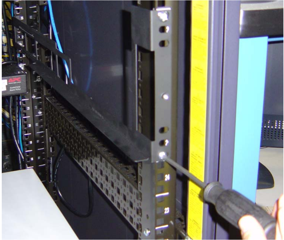
Figure 1-4: Attaching Rails from the Front
