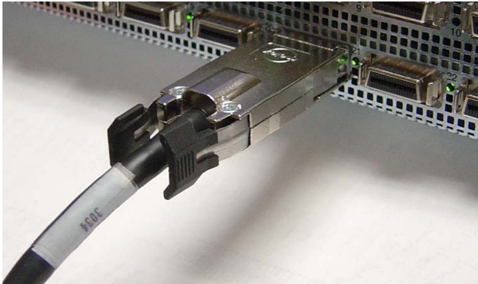
Figure 1-9: Fully Installed IB Cable with Pinch Connector
