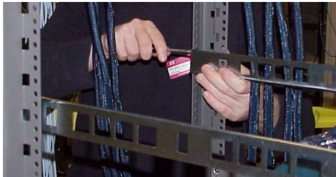
Figure 2-4: Secure Rail Bracket to Rack with Screws
