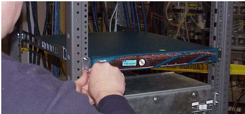
Figure 2-6: Secure Switch with Screws through the Front of the Rack
