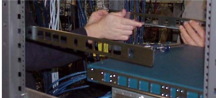
Figure 2-3: Holding bracket against inside of rack
