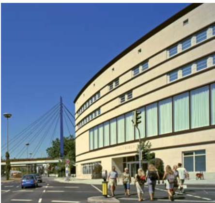
City Library, City of Pforzheim
