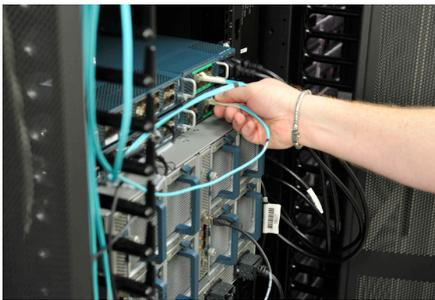
Hubs for the core network were installed at ten locations on the grounds of the Port of Hamburg and connected using optical waveguides. The various LANs were then docked onto these. This allows employees to communicate with each other and exchange documents regardless of where they are and what device they happen to be using.
